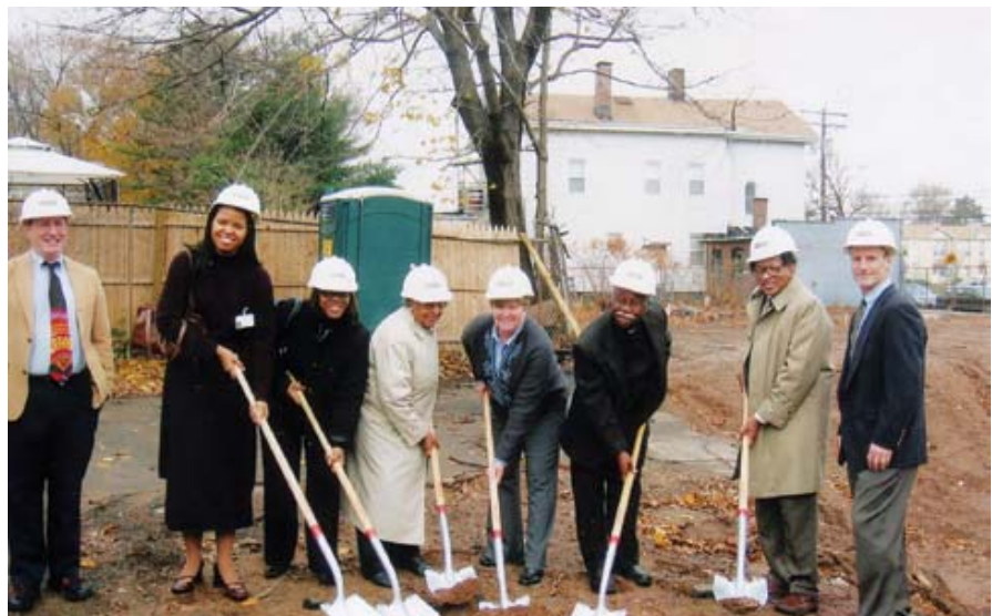
Josephine Gray (fourth from left) joins others in breaking ground on the new senior housing facility named after her. The Community & Economic Development Clinic has been helping St. Luke's Senior Housing to make the building a reality.
