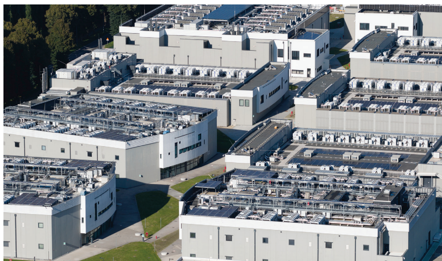
One of many data centers increasing demand on the electric grid
